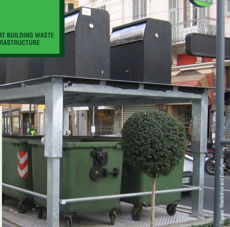
Raised Platform showing Underground Bins
