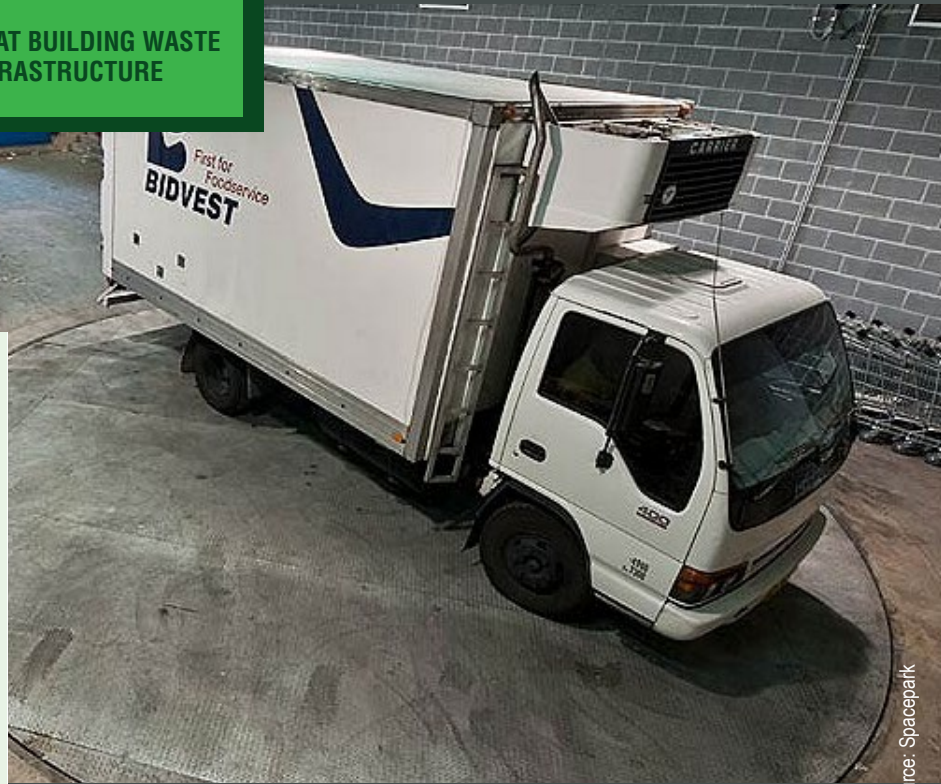
Truck Turntable in Loading Dock
