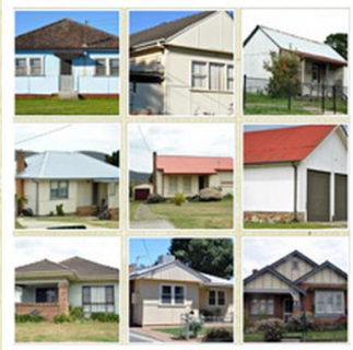
HOUSES WITH ASBESTOS
